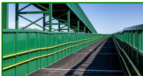
The new bridleway bridge at Lindsells Level Crossing
