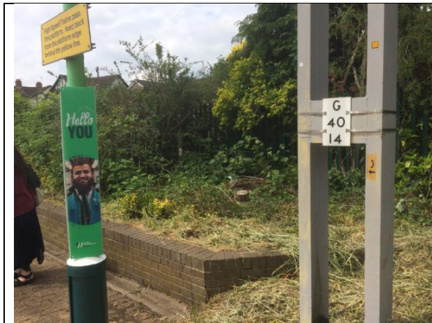
At point H on fast line platform looking south-westwards to point J
