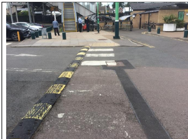
Looking westwards from point C towards point D across station car park entrance
