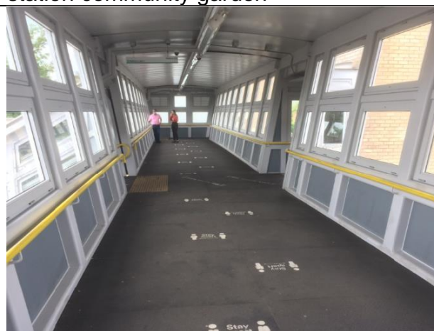
Looking westwards along northern footbridge
