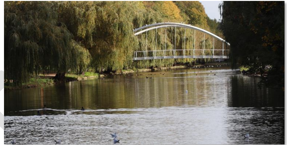
River Ouse through Bedford Embankment – Ben Woodhouse
